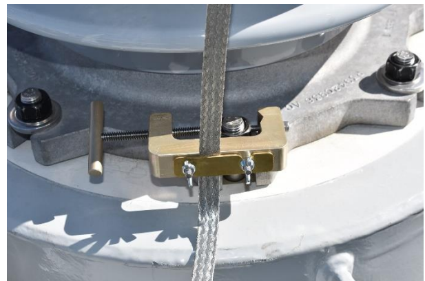
Earth connection to the ground clamp
